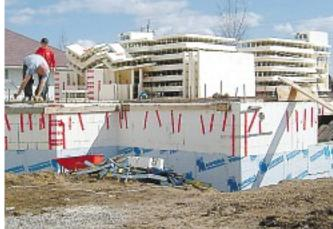
Super-solid construction of Dabrro's Wetaskiwin showhome includes poured concrete and rebar.
