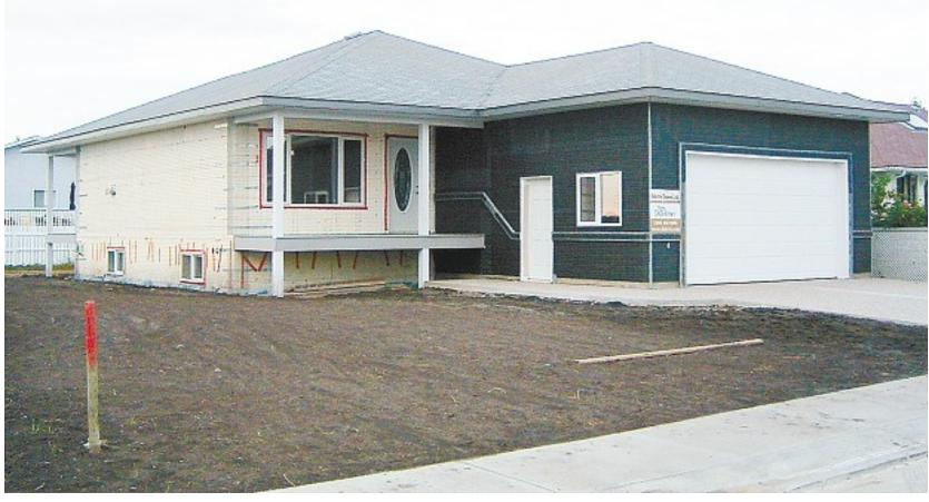
Exterior walls include cement, insulation and rebar.
